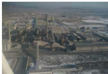
Korea Magnesia Clinker Industry Group's extensive plant at Danchon, North Korea. The group has in total 74 shaft kilns and two rotary kilns with a combined DBM capacity of 1.2m. tpa.
