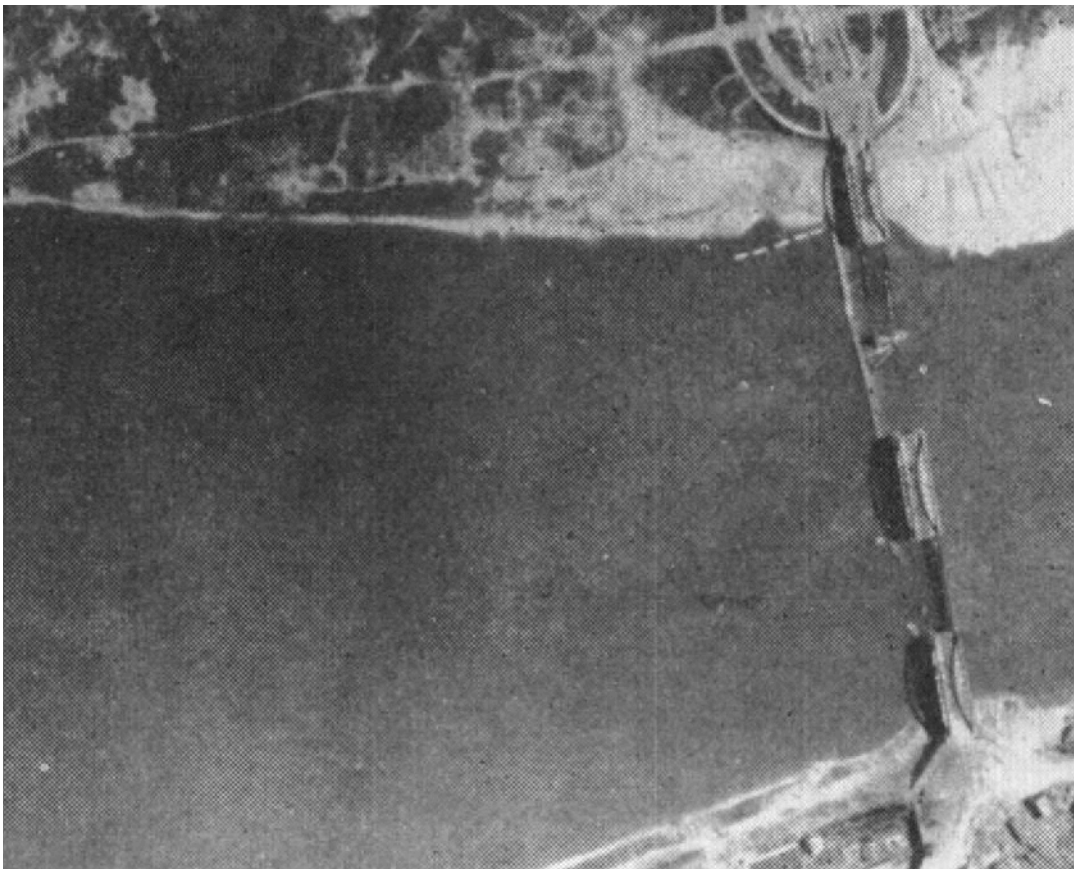
Photo #7: Taken on 11 August 1950 this photo shows that additional damage has been done to the structure of highway bridge. While the pontoon bridge has either been damaged or temporarily broken apart to simulate damage. Note the pontoon section floated to the northern bank. (USAF)
