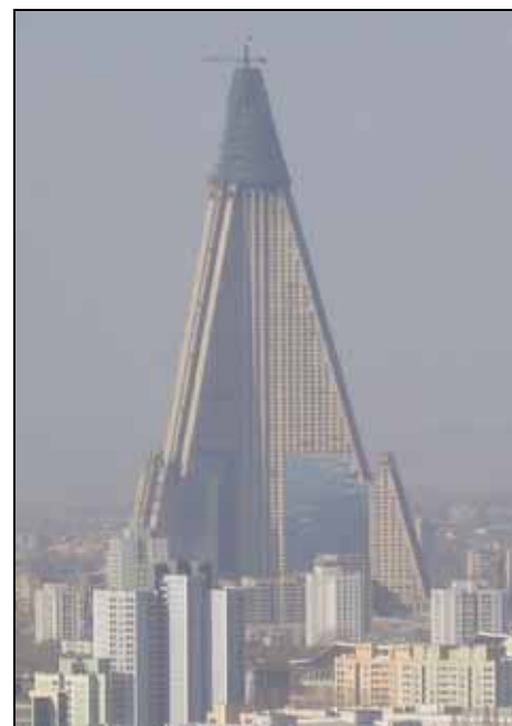
Progress work continues on Pyongyang's landmark 105-storey Ryugyong Hotel in cooperation with Orascom's construction arm.
