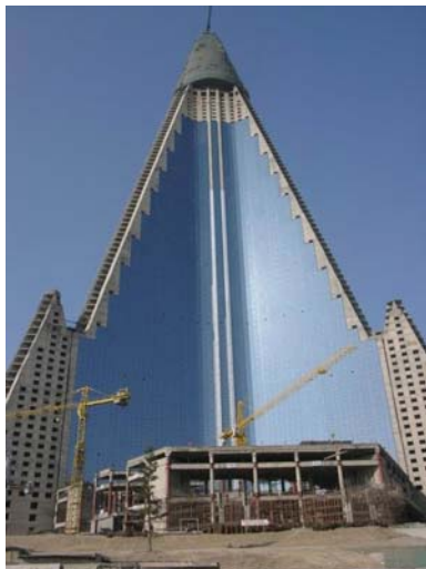
Photo: work on the Ryugyong Hotel
