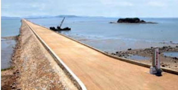
View of Breakwater No.3 [Photo:KCNA]
