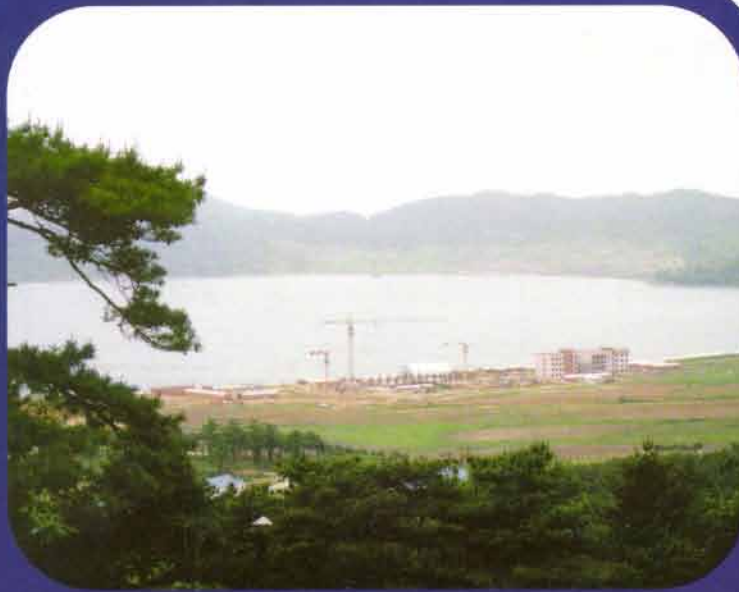
View of Pipa Island and the Emperor Group (HK) hotel construction site
