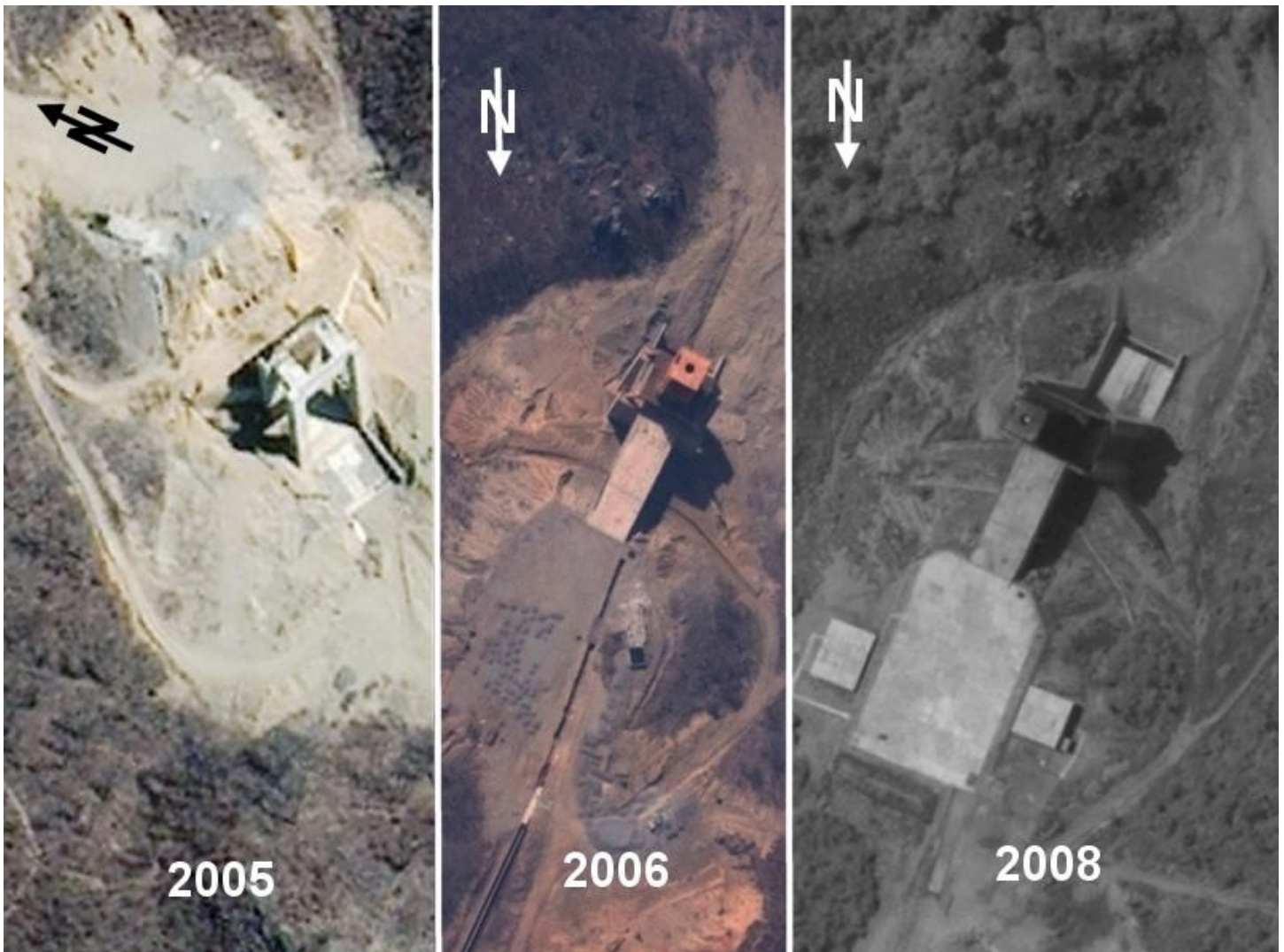
Figure 6. Construction sequence at the engine test stand. (credit: Left image- GeoEye. Center and right images - DigitalGlobe)
