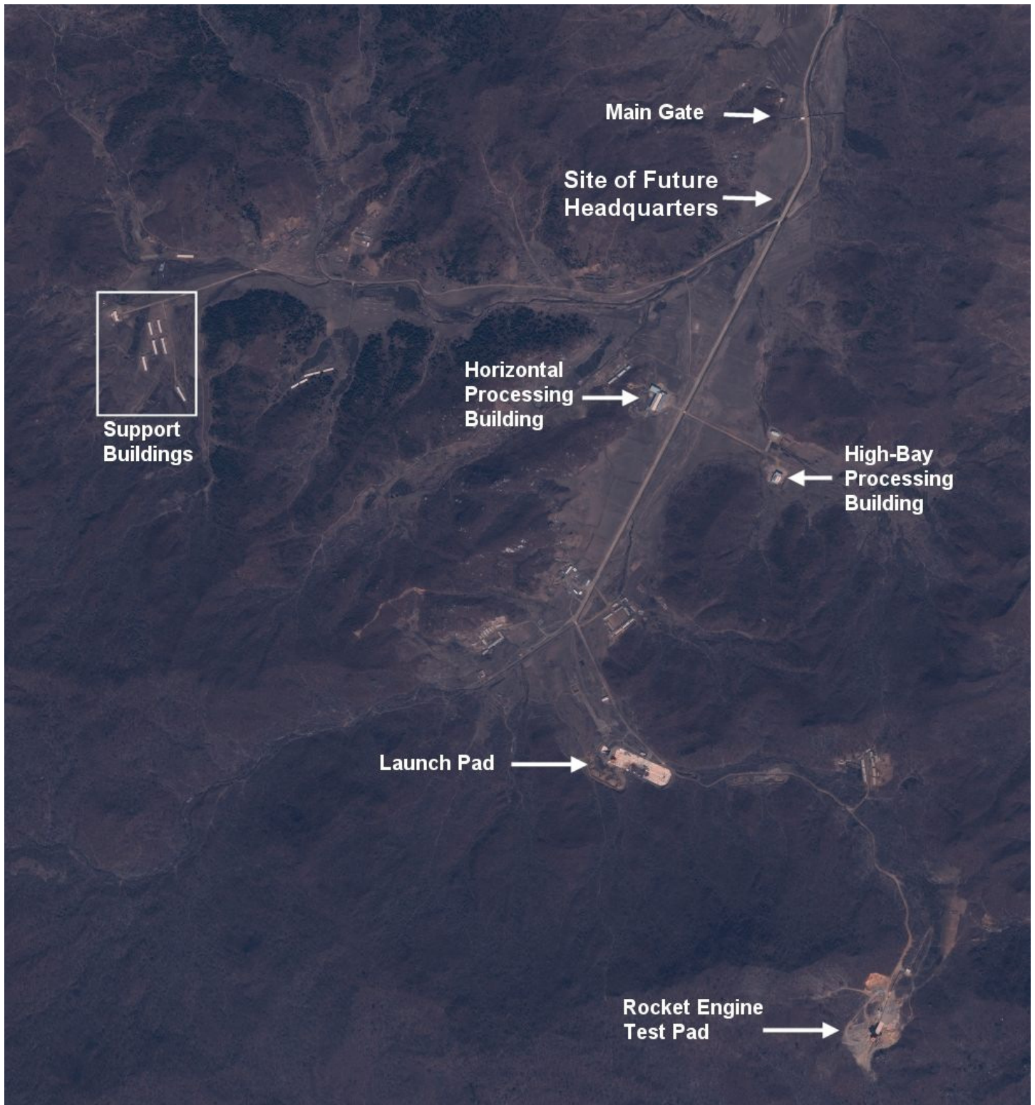
Figure 4. Imagery from 1 April 2006, Shows the progress of construction activity. (credit: DigitalGlobe)
