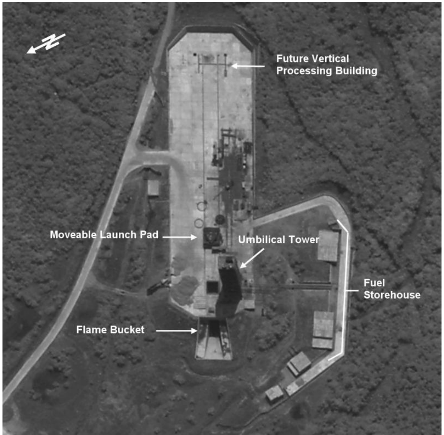
Figure 5. Overview of the Launch Facility as of 22 June 2008. (credit: DigitalGlobe)
