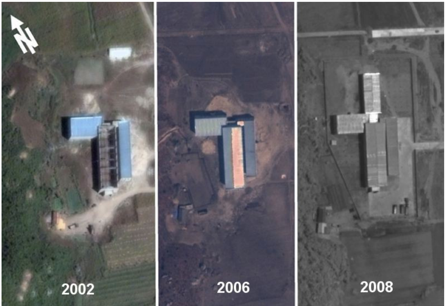
Figure 8. The horizontal processing building at Pongdong-ni. (credit: DigitalGlobe)
