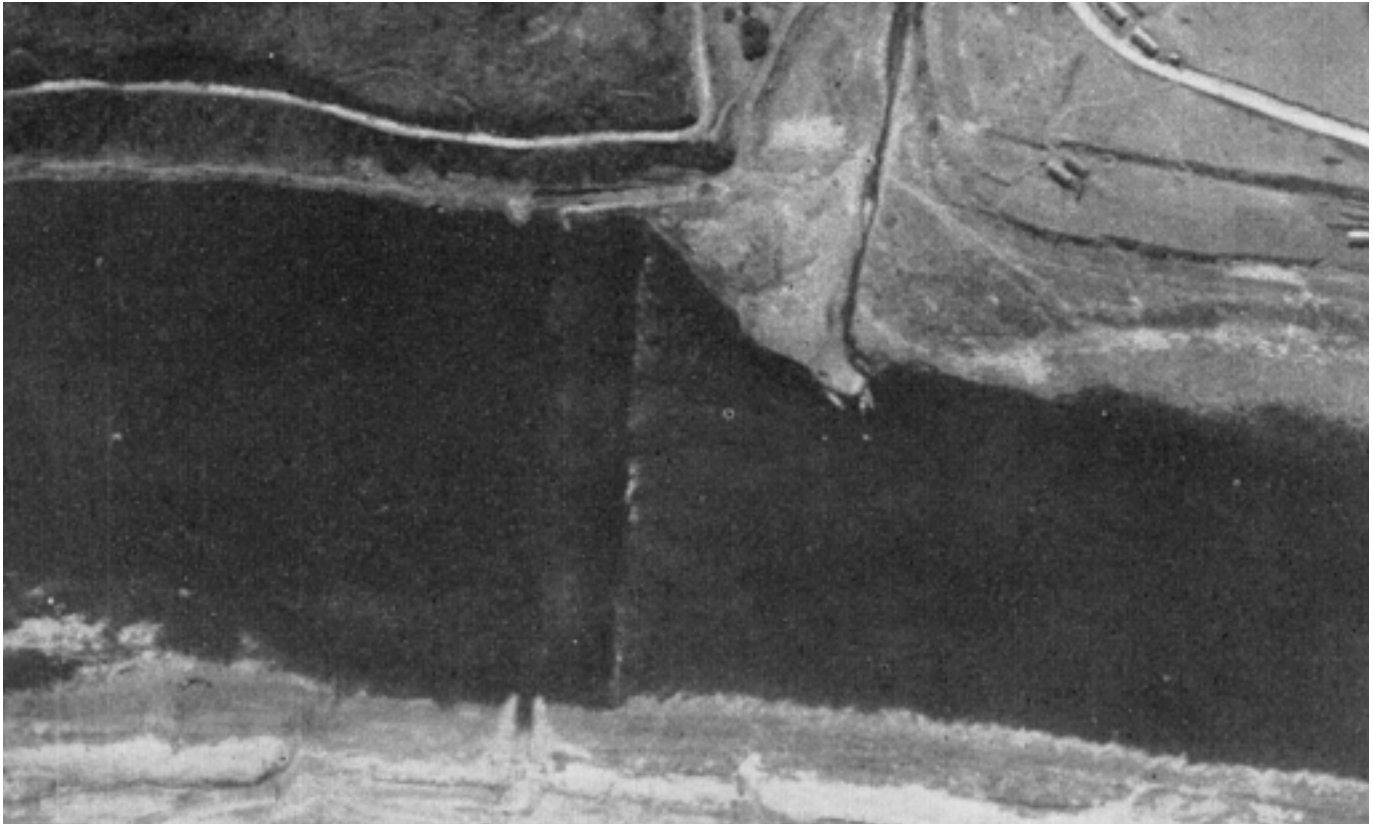
This photo, taken on 18 April 1951, shows one of the many underwater crossing constructed by the KPA. This one is 5 km southwest of Manpojin. Sandbags were piled on river bottom until a structure 4.5 m wide was raised to within .6 m of the surface. Immediately downstream (to the right in the photo) of the crossing the KPA hastily constructed a "leaky" dam. Its purpose was to raise and calm the waters upstream at the crossing. (USAF)
